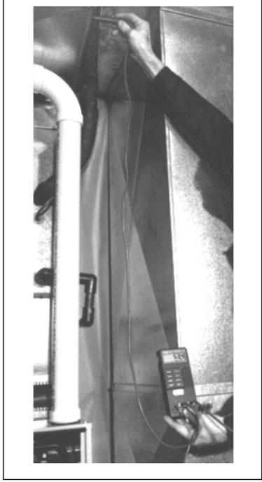
INSTALLER MUST ADJUST THE TEMPERATURE RISE TO THIS "MIDDLE" POINT AS CLOSELY AS POSSIBLE. ALSO, THE TEMPERATURE RISE SHOULD NEVER BE ABOVE OR FALL BELOW THE STATED RANGE. DOING SO COULD CAUSE DAMAGE TO THE HEAT EXCHANGER OR INTERMITTENT OPERATION WHICH COULD CAUSE INJURY OR DEATH AND WILL VOID THE MANUFACTURER'S WARRANTY FOR THIS PRODUCT.
