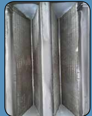
10 year old air conditioning coil with whole-house air cleaner
