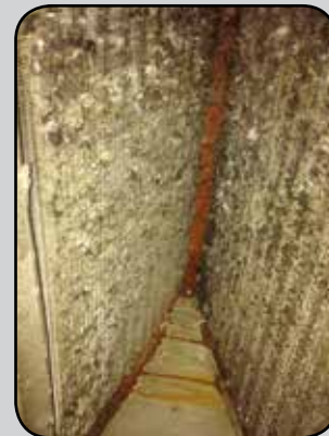
10 year old air conditioning coil without whole-house air cleaner
