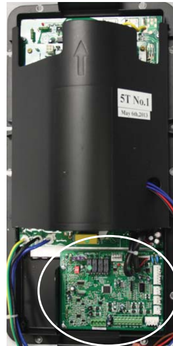
Fig. 17 – AOC (Application Operational Control) Board
