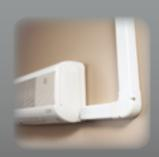
DiversiTech recommends attaching the base to the wall or ceiling and the line sets to the system every 15" to allow for the system to carry the full weight of the line sets.
