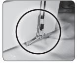
**Step 7:** Using the ratchet end of the ratchet strap, attach each strap to the eye bolts above the unit. If additional slack on the rope is needed, push the trigger on the ratchet end of the strap up and feed the rope through as needed.
