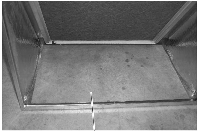
BOTTOM BLOCK OFF PLATE REMOVED
