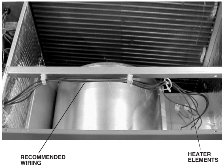
FIGURE 5 HEATER KIT INSTALLATION
