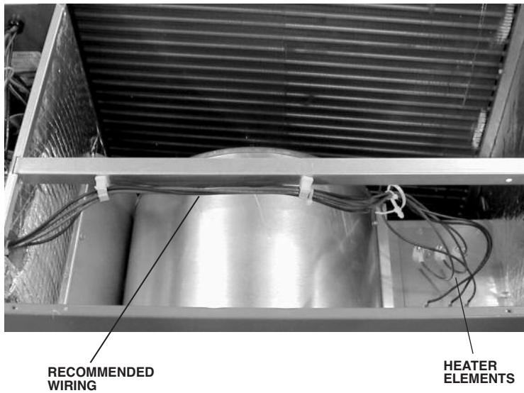
FIGURE 5 HEATER KIT INSTALLATION
