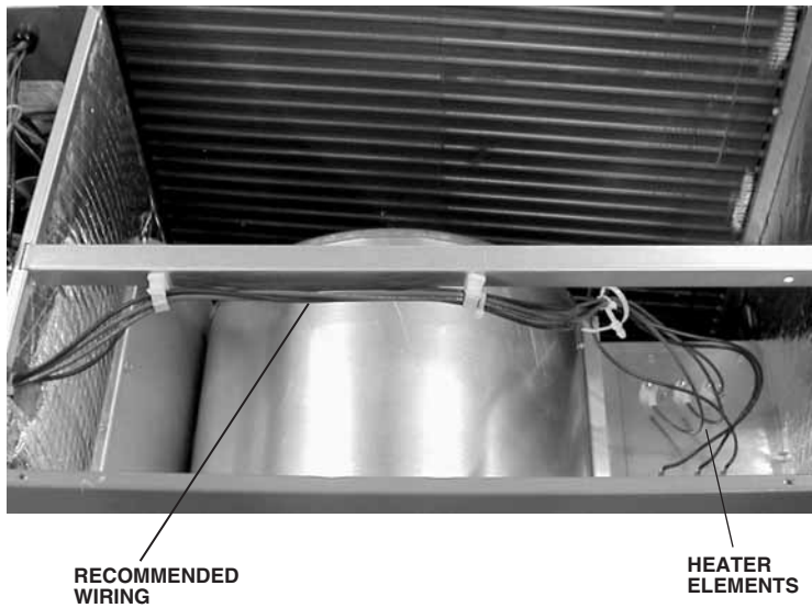
FIGURE 5 HEATER KIT INSTALLATION
