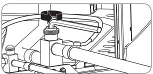
After adequate evacuation, open both service valves by removing both brass service valve caps with an adjustable wrench. Insert a 3/16" [5 mm] or 5/16" [8 mm] hex wrench into the stem and turn counterclockwise until the wrench stops.
