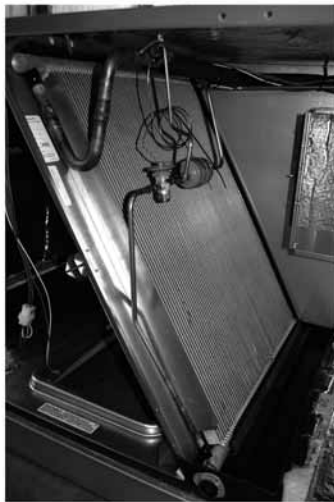
Evaporator Coil/Filter Access
