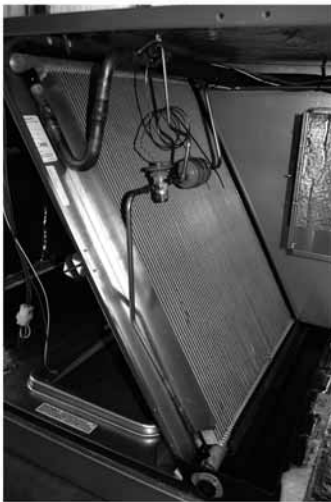
Evaporator Coil/Filter Access
