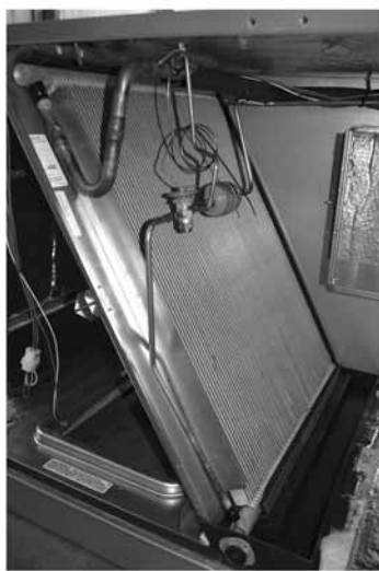
Evaporator Coil/Filter Access
