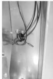
Discharge Air Sensor
