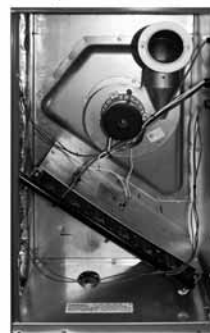
Heating Compartment Access
