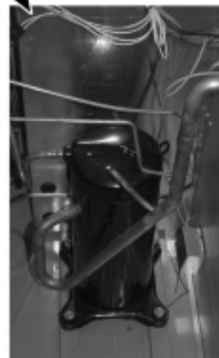
Compressor Access (3 to 5 Ton [10.6 to 17.6 kW] Models)
