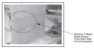
9. Tilt the coil assembly forward. (Note: Depending upon the amount of slack in the refrigerant lines, the system may have to be evacuated and the suction and liquid line of the air handler may have to be uninstalled from the system in order to prevent damage to the refrigerant lines which could result in a total loss of refrigerant)
