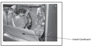
6. Remove the 3 sheet metal screws which attached the blower to the blower shelf located in the air handler control box. (3/8" Socket)
