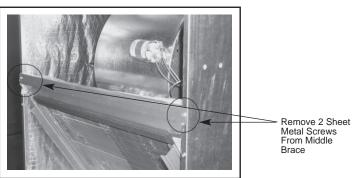
8. Remove 4 sheet metal screws (2 on each side of the air handler)
