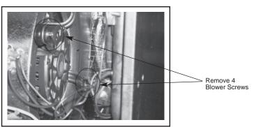
11. Remove the motor assembly from the blower housing by sliding the motor shaft out of the blower hub.
