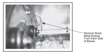
8. Remove the 3 sheet metal screws which attached the blower to the blower shelf located in the air handler control box. (3/8" Socket)
