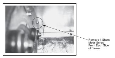
11. Remove the 3 sheet metal screws which attached the blower to the blower shelf located in the air handler control box. (3/8" Socket)
