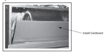
6. Remove the top plate of the air handler by removing the 6 sheet metal screws attaching the plate to the top of the air handler. (1/4" Socket)
