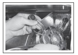
12. Remove the motor assembly from the air handler.
