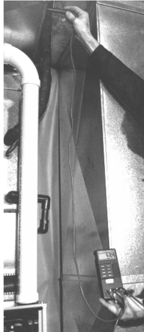
FIGURE 49 TEMPERATURE RISE MEASUREMENT
