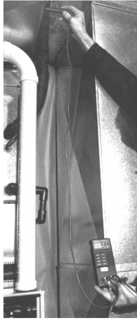
FIGURE 49 TEMPERATURE RISE MEASUREMENT
