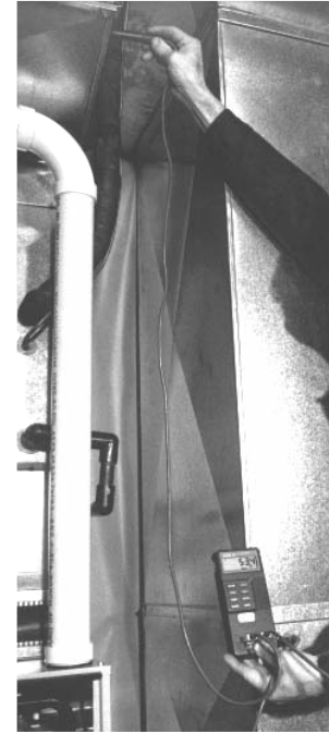
FIGURE 49 TEMPERATURE RISE MEASUREMENT
