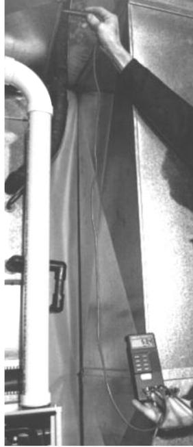
INSTALLER MUST ADJUST THE TEMPERATURE RISE TO THIS "MIDDLE" POINT AS CLOSELY AS POSSIBLE. ALSO, THE TEMPERATURE RISE SHOULD NEVER BE ABOVE OR FALL BELOW THE STATED RANGE. DOING SO COULD CAUSE DAMAGE TO THE HEAT EXCHANGER OR INTERMITTENT OPERATION WHICH COULD CAUSE INJURY OR DEATH AND WILL VOID THE MANUFACTURER'S WARRANTY FOR THIS PRODUCT.
