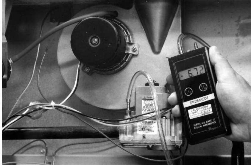
FIGURE 16 TYPICAL HOSE CONNECTION TO LINE PRESSURE TAP
