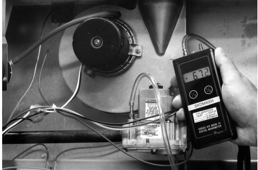
FIGURE 16 TYPICAL HOSE CONNECTION TO LINE PRESSURE TAP
