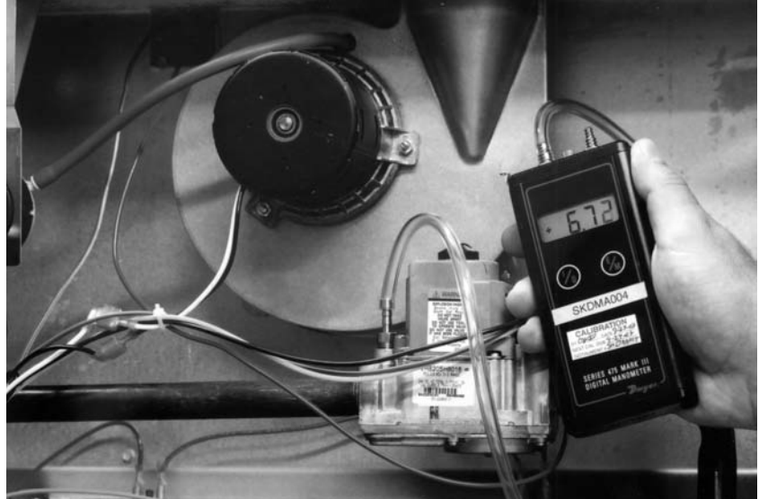
FIGURE 16 TYPICAL HOSE CONNECTION TO LINE PRESSURE TAP
