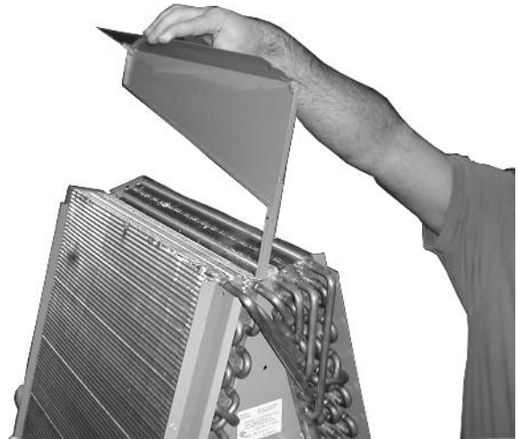
FIGURE 9 ROTATE DRAIN TROUGH
