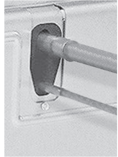
FIGURE 9 COMPLETED REFRIGERANT CONNECTION ASSEMBLY
