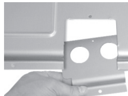
FIGURE 14 INSTALLING CONDENSATE BLOCK-OFF PLATE
