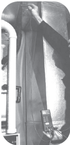
FIGURE 48 TEMPERATURE RISE MEASUREMENT
