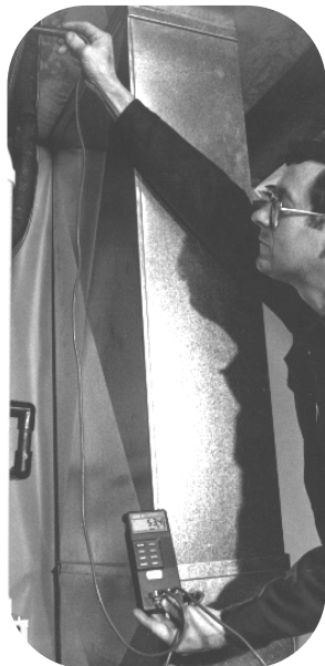
FIGURE 48 TEMPERATURE RISE MEASUREMENT
