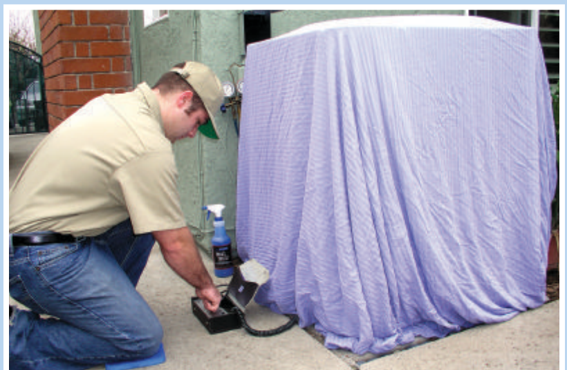
Cover the condensing unit (or section on a package unit) to pick up any refrigerant drift. The cloth barrier prevents air dilution.
