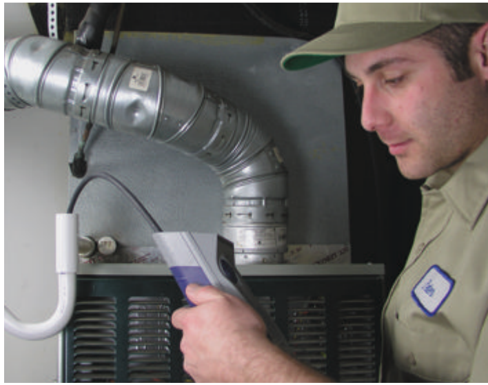
Sniff the outlet of the condensate drain pipe to confirm or rule out an evaporator leak.
