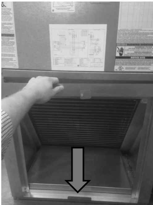
INSERT NEW FILTER RACK
