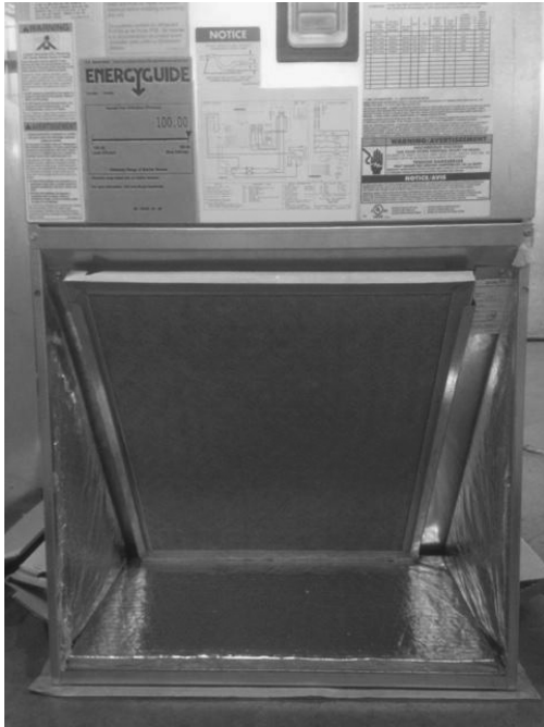
REMOVE EXISTING AIR FILTER
