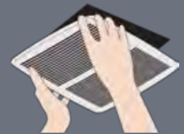
4. Install new grille
