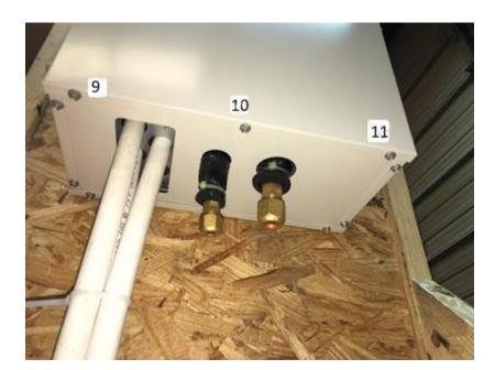
10. Install enclosure top(item #5) to the enclosure with four screws provided.
