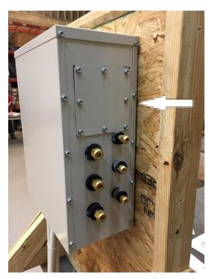
12. Use field supplied silicone sealant to seal around line set locations. Ensure sealant is completely sealing line set insulation and enclosure Line Set Side (item #3). This is required for all outdoor applications.
