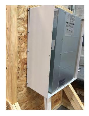
8. Complete all wiring and piping to branch box at this point. Refer to Branch Box installation instructions for Dip switch settings and addressing.
