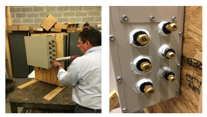
13. Complete all line set and electrical connections as required by branch box manufacturer.
