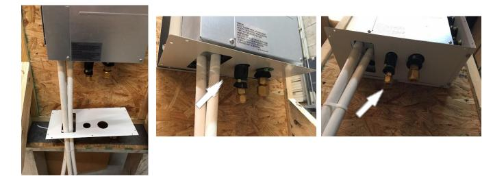
5. Attach the enclosure line set side (item #3) to the back panel and bottom panel.
