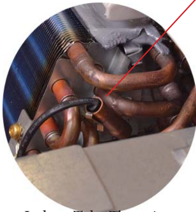
Indoor Tube Thermistor
