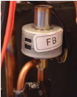
Electronic Expansion Valve
