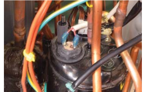
Compressor Overload
