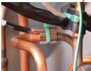
Exhaust Temp Sensor
