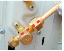
Apply pressure to hold tube against male flare body while hand tightening and then mark the starting alignment before final turn. If necessary, maintain pressure on tube until nut tightening prevents tube drift. TURN
