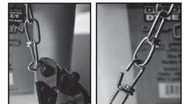
Cut with Duro Dyne Cable Cutter
