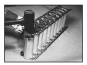
Assembly is ready to be inserted into the duct. Fasten to duct wall per SMACNA recommendations.
