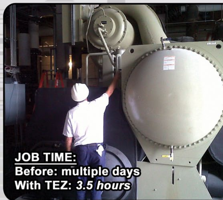
Above: This 2,000 ton chiller was pulled from atmosphere to 1,000 microns in only 3.5 hours... instead of days with a belt-driven pump.
