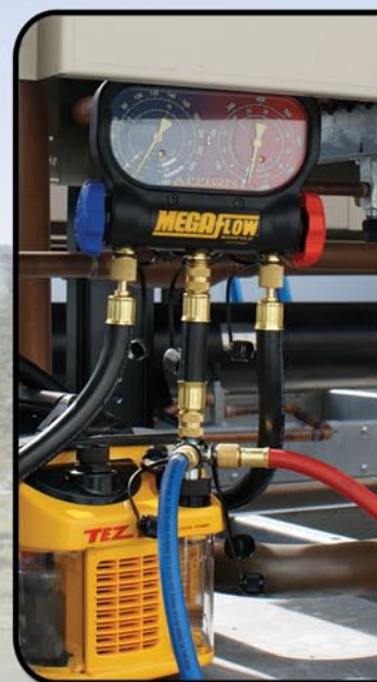
Above: At a large refrigeration job, a Bohn 30HP chiller went from 1000 microns to 500 microns in just 4.25 hours... much faster than a belt-driven pump.
