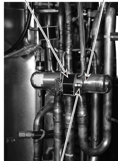
4-way valve coil (21S4)
