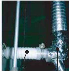
Figure 53: Properly Insulated Condensate Drain Piping.
