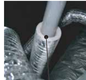
Figure 53: Properly Insulated Condensate Drain Piping.
