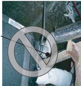
Figure 54: Condensate Drain Piping Should Not Include Sharp Bends.
