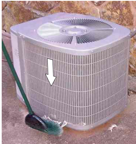
Figure 2: Cleaning with a broom.
